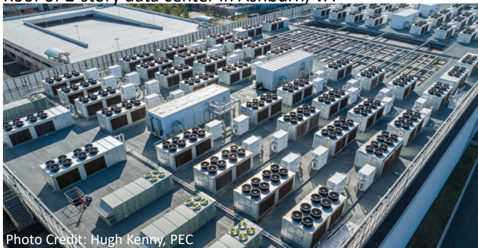
Roof of 2-story data center in Ashburn, VA
