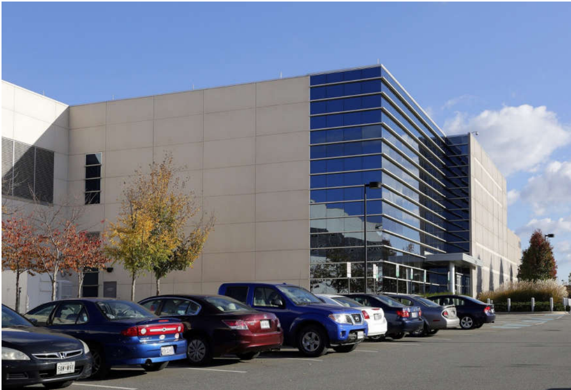
Digital Reality colocation data center with conference and work space
