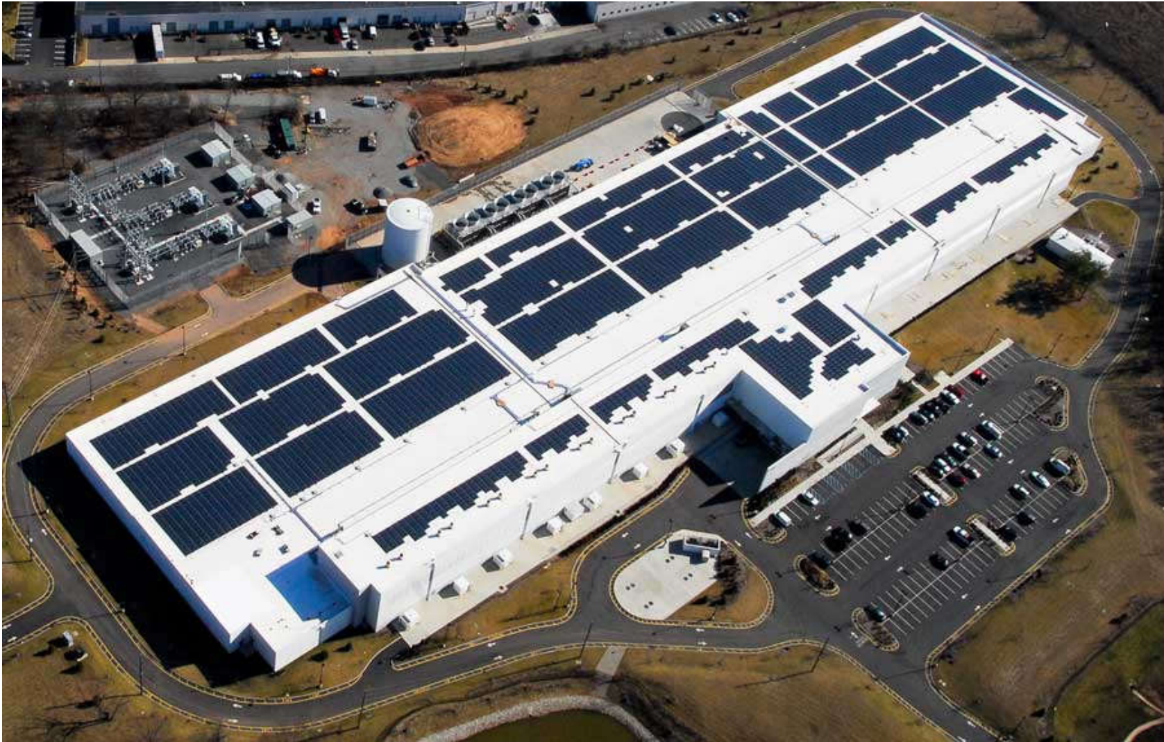
DuPont Fabros NJ1 data center in Piscataway, New Jersey (now owned by QTS)
