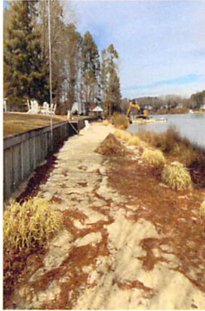
View of southern waterfront along Piankatank River.
