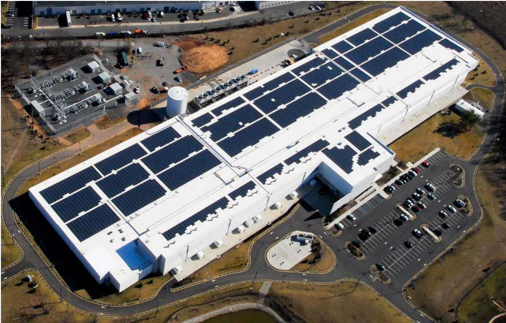
DuPont Fabros NJ1 data center in Piscataway, New Jersey (now owned by QTS)
